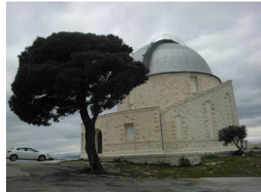
The historical building of the institute at Penteli mountain
